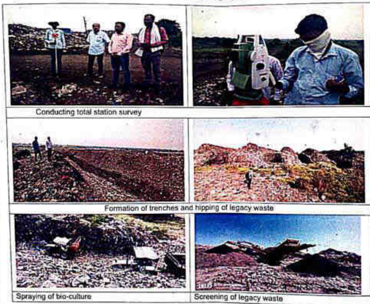
Figure 2-3 : Phases of Bioremediation and Biomining of legacy waste Sukhali compost depot
